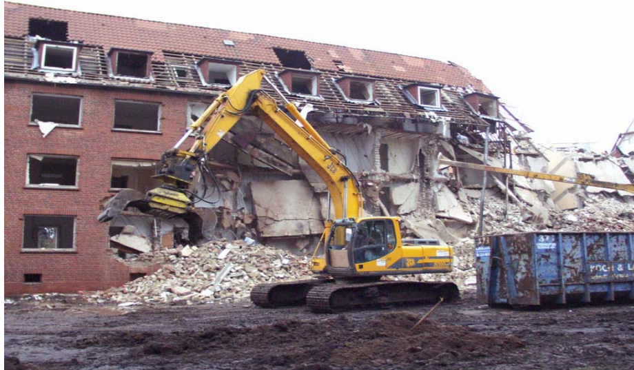
Start of demolition July 2000
