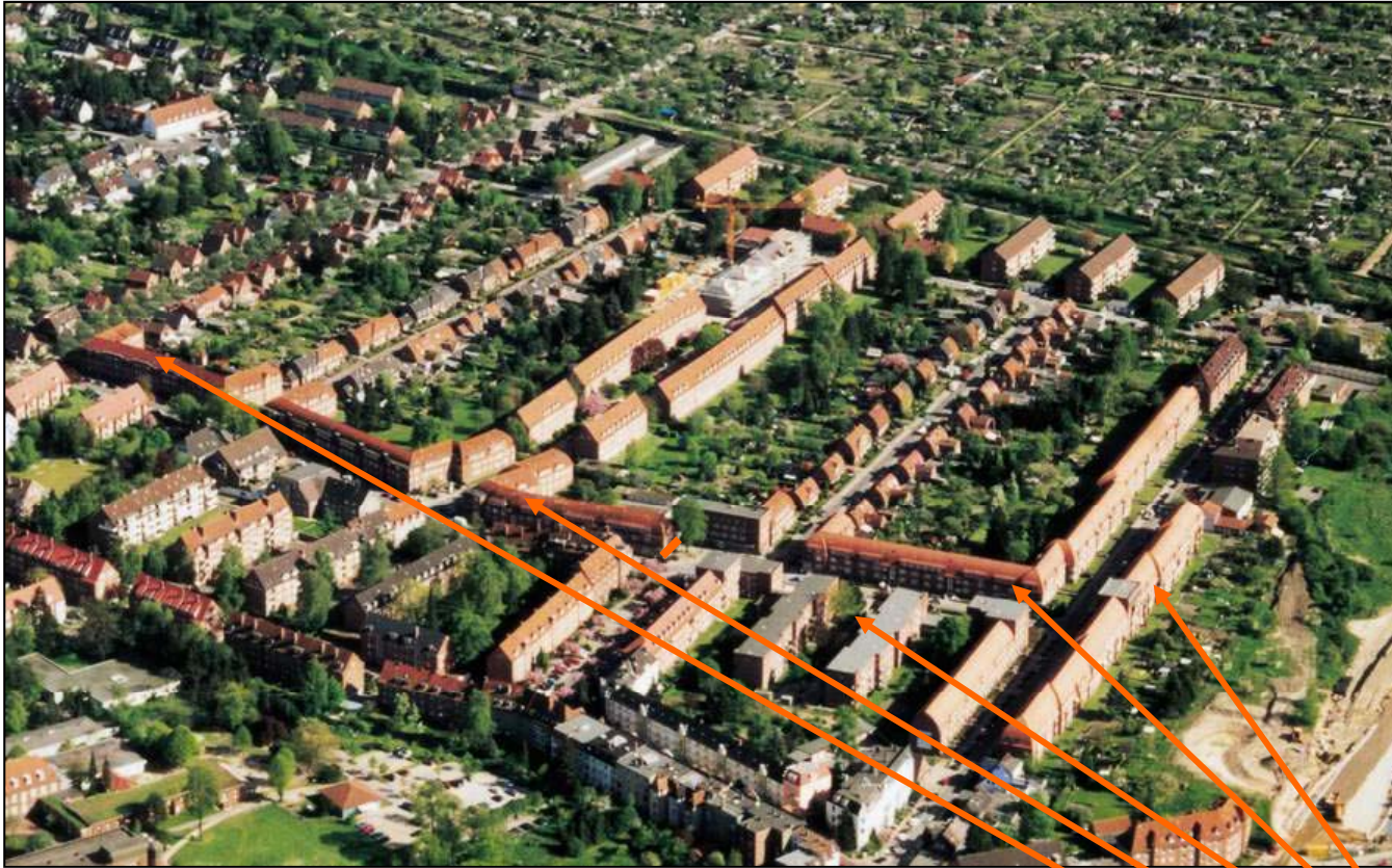
Refurbishment of the buildings from the 1920`s (475 flats)
